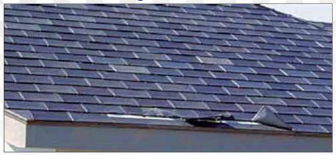
Dark gray colored stainless steel tile roof in the Bahamas. After a direct hurricane hit at 160 miles an hour (256 Kmph), this roof suffered only a minor damage as can be seen in the picture above. All of the surrounding homes lost their roofs. This is a living proof of the capability of stainless steels to resist calamities. In Japan, large stainless steel storage tanks for water have been made to withstand earth quakes to ensure water supply to the stricken people.
